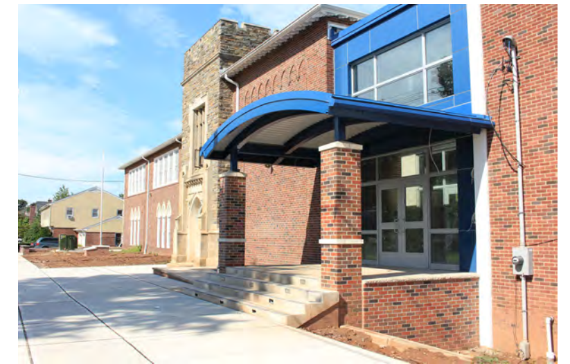
FINISHING TOUCHES: The new First Street entrance of the renovated Wood-Ridge Intermediate School.
