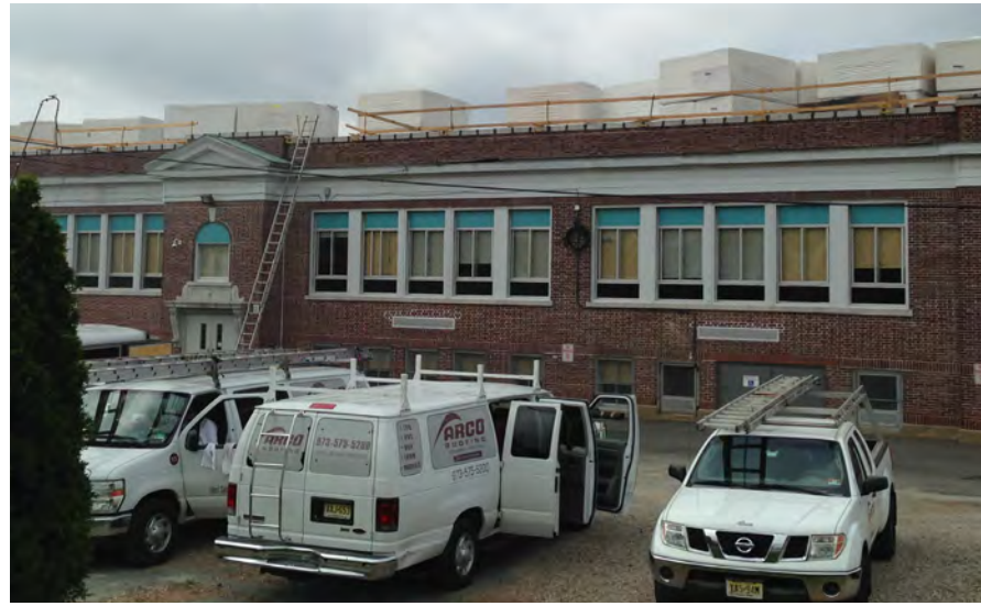
Wood-Ridge High School is receiving a new roof this summer.
