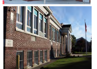
A comprehensive series of improvements at Doyle, Ostrovsky and Wood-Ridge High Schools will bring enhanced security, comfort, and educational resources to the three buildings during 2015-2016.
