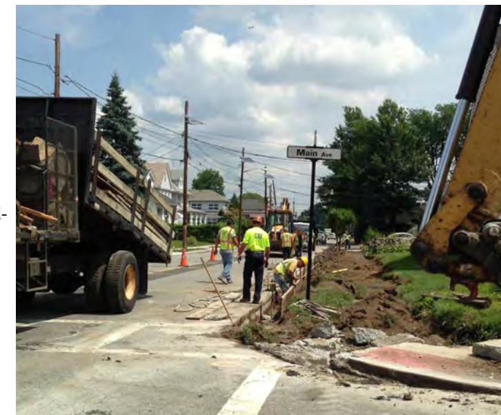
(Above) New curbs and sidewalks being installed on Valley Boulevard; (Below) Traffic calming measures installed by the Borough along Highland Avenue.
